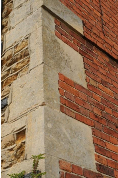
Left: Dressed (Lincolnshire) limestone quoins (on a larger costlier house) at the junction between a front (undressed limestone/ironstone wall and a red brick side wall.
