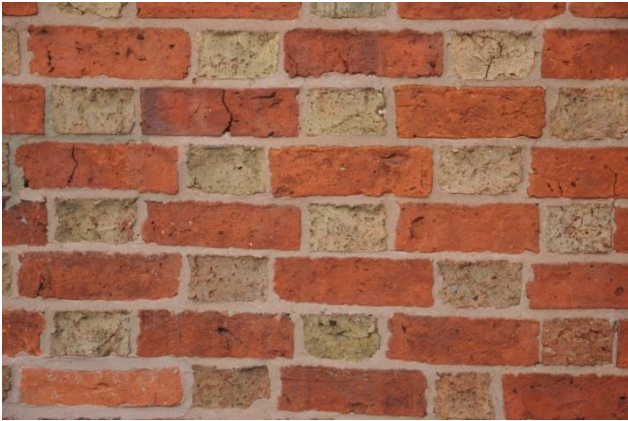
Left: A “Chequerboard” wall on a house using red and cream bricks laid in an alternating header stretcher pattern on each course, with flush pale grey/brown mortar & pointing.
