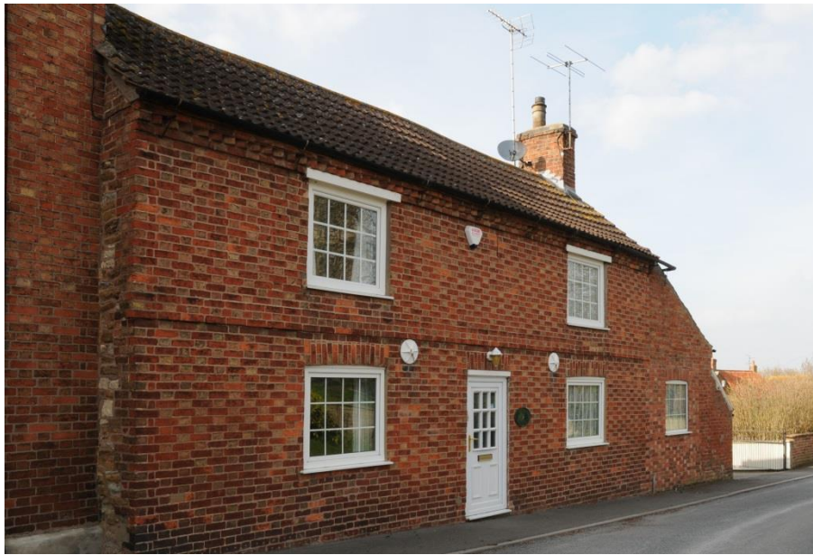
4: C18 cottage & outbuilding. String course & dentil under eaves. Concrete interlocking tiles, 2 chimneys. New door/windows but original openings.
