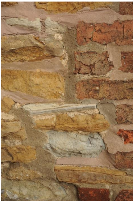
Left: Roughly tied in jointing between unsorted (Ironstone, Limestone & Blue Lias) stone wall and an old red brick wall
