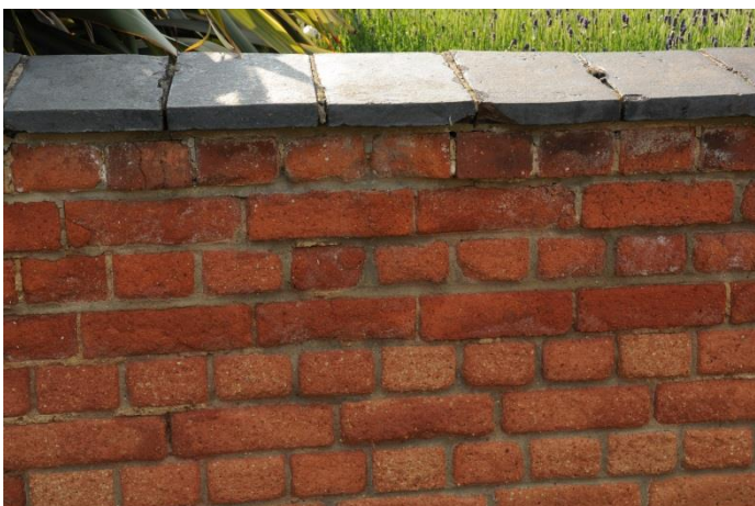
Left: C19/20 garden wall, red brick English Garden Wall bond; alternating header & stretcher courses. Flat blue clay coping stones with overhang. Recessed/worn pointing.
