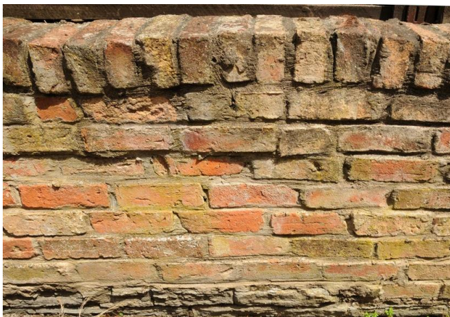
Left: Low brick wall with informal coursing using old mixed red bricks and brick on edge coping
