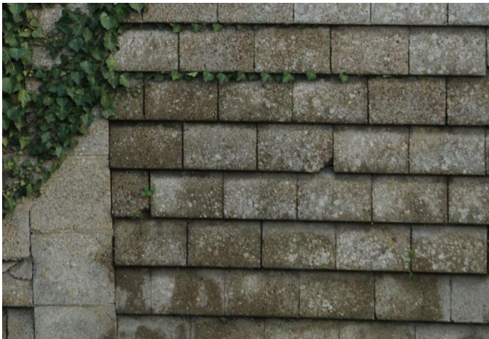
Left: Tile hanging (the only local example) using modern regularly shaped blue/grey concrete tiles. Pillar to left appears to be concrete or granite not to be encouraged.
