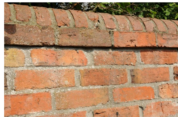
Traditional red brick garden wall, flush pointed. Coursing is Flemish Bond; headers every 6 th course. Semi-circular coping bricks (manufactured) on wider stretcher course.
