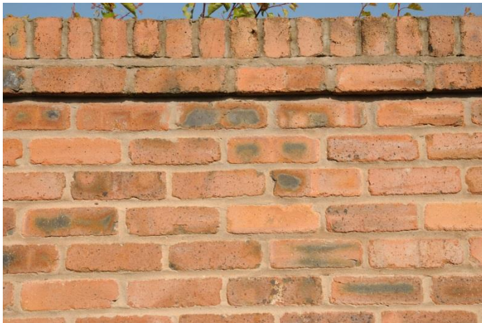
Left: Recent pale red brick garden wall using metal ties with no coursing, under brick on edge coping laid on widened stretcher course, with pale mortar and flush pointing.
