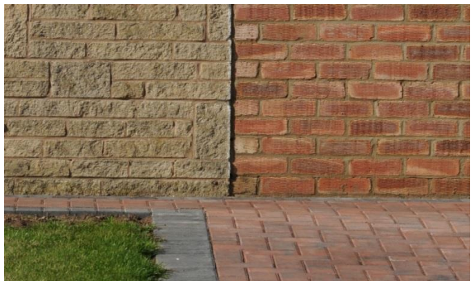
Above right: Imitation stone and red brick used on some of the bungalows with block paving.
