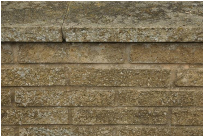
Left: Artificial stone (concrete) grey block wall regular size/shape similar coping stones/slabs. Bucket handle pointing. (This is around the church on Church Street and is inappropriate).
