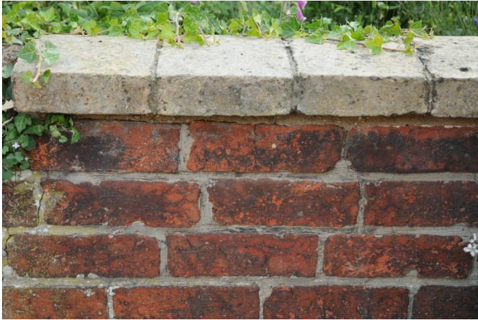
Left: Older red brick garden wall with coursing likely, but not visible, under dressed limestone coping slabs. Slightly recessed pointing with grey mortar.
